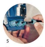
The overall insulation of the cable must be inside the housing to guarantee proper sealing of the cable gland
