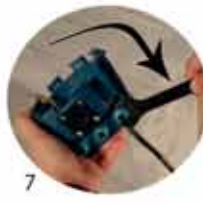
7 The female part must be properly tightened with a spanner or similar
