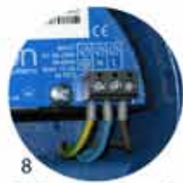
8 All three power supply conductors must be properly tightened.
