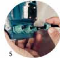
5 The overall insulation of the cable must be inside the housing to guarantee proper sealing of cable gland
